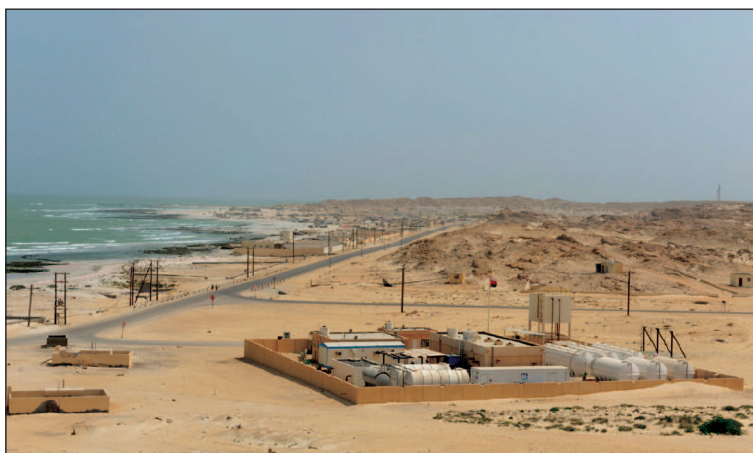
Figure 4: Forward osmosis based desalination plant, Oman.
