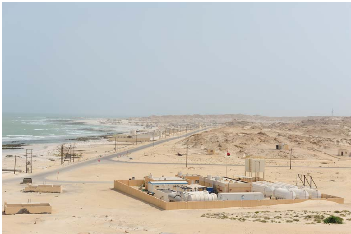
Figure 4: Forward osmosis based desalination plant, Oman
